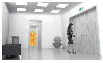
If a fire is detected by the fire detection and fire alarm system, the pathfinder luminaires can safely guide the escaping people from the danger zone. To this end, the alternative 2nd escape route is revealed. The indication of the 1st escape route in the danger zone is now not visible.
