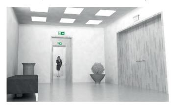
During normal operation, the pathfinder luminaire indicates the designated 1st escape route. Indication of the alternative 2nd escape route is not visible.
